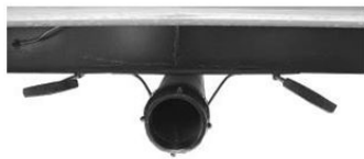
Black/Grey tank drain & valves
